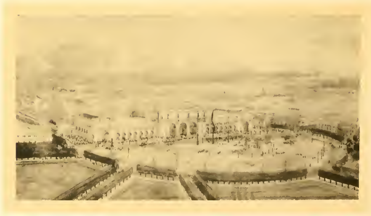
XXVI. THE PLAZA AND UNION STATION, WASHINGTON, BEGUN IN 1902.
